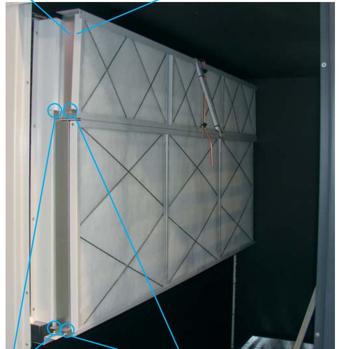
Tabs for displacement of the opacimetric filters
