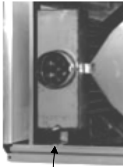
Threaded condensate drain union
